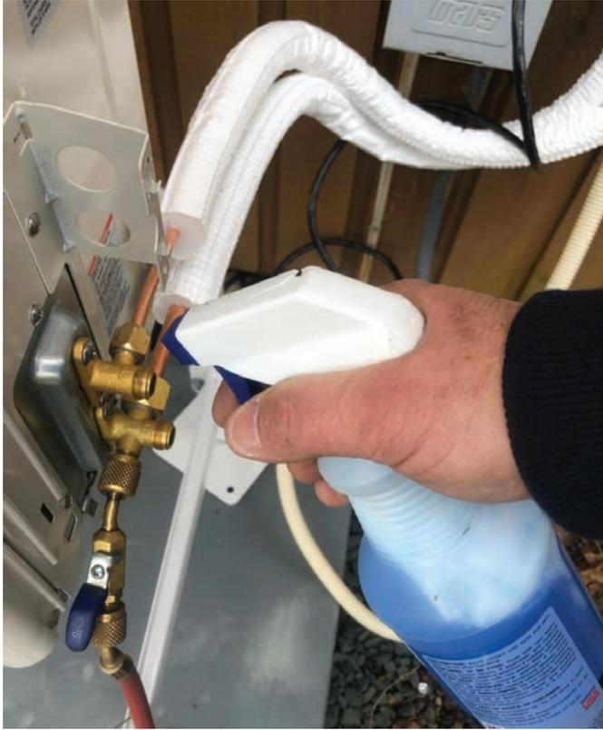
While the line sets are filled with high-pressure nitrogen, apply a leak-testing solution to all flares.
